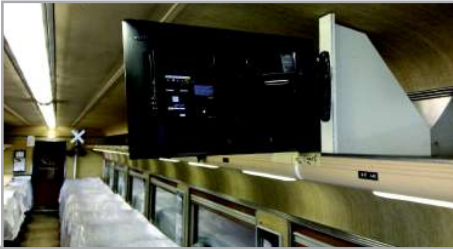
Mounting each display was especially challenging in these railroad cars. Mounts were custom fabricated, with prototypes being tested. This mount also allowed the displays to swing and face the other direction, if needed.
